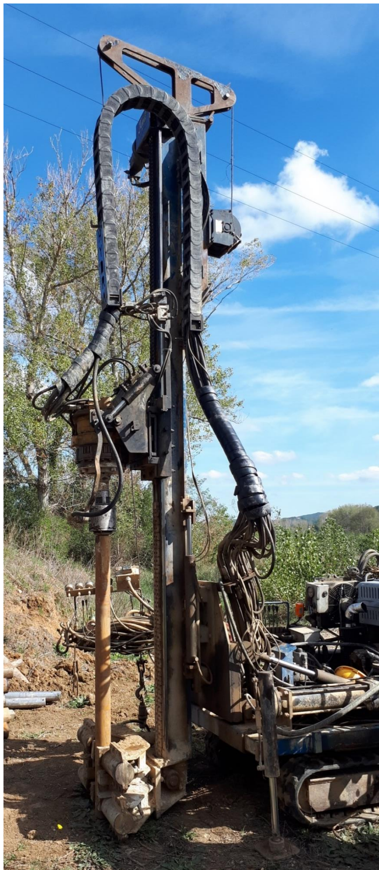
Drilling of a piezometer.
