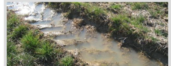
Evidence of soil compaction
